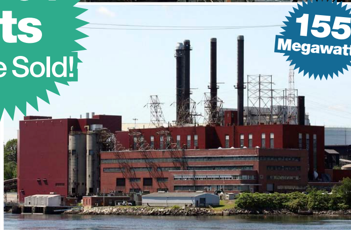
155 MW Plant in Portsmouth, NH
