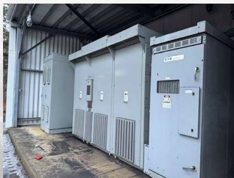
Eaton Cutler Switchgear , Approx 2000 Amp, with 12 Breakers, 800 Amp, Approx. 8 Ft x 7 Ft x 8 Ft, (Lot 328)
