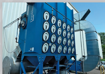
75 HP Torit Model DF04-48 Downflo Oval 48-Cartridge Dust Collector
